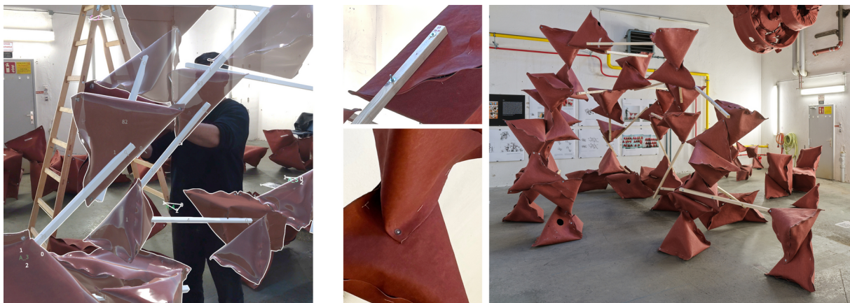
Figure 8: AR-guided assembly (left), joint details (middle), and final installation (right).
