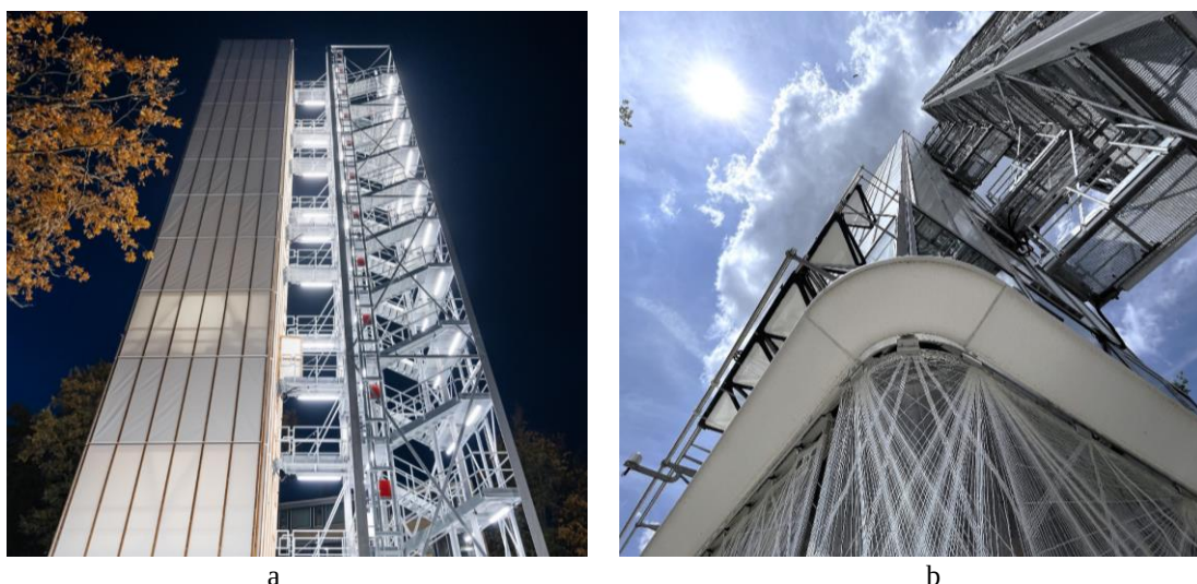
Figure 5: D1244 after erection in 2021 (Photo: René Müller) (a) and with the first integrated facades in 2025 (Photo: ILEK) (b).
