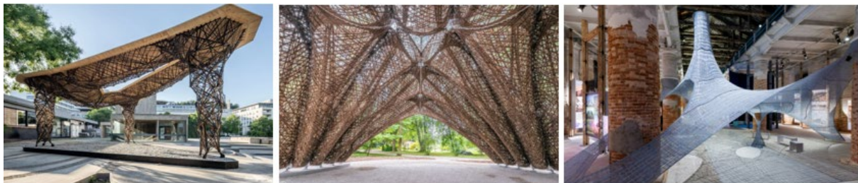
Figure 4: State of the art in flax-fiber based architectural investigations with the focus on fiber performance, aesthetics and exposure. Left to right: ICD-ITKE Research Pavilion 2024, livMats Pavilion 2024, Necto 2025.
