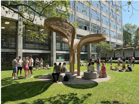
Figure 1: TimberTwist - Wood in Rotation: Full-scale bending-active canopy showing three zip-bent timber ribs, pre-tensioned high-tensile membrane, and support/anchorage points. Left image: Rendering photograph of the pavilion on the University of Stuttgart city center campus. Right image: Exploded schematic of the ribs as zipper-composite elements created by CNC-milled kerf patterns.
